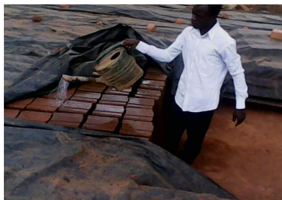
Fig. 7. Curing and storage of compressed laterite interlocking blocks
