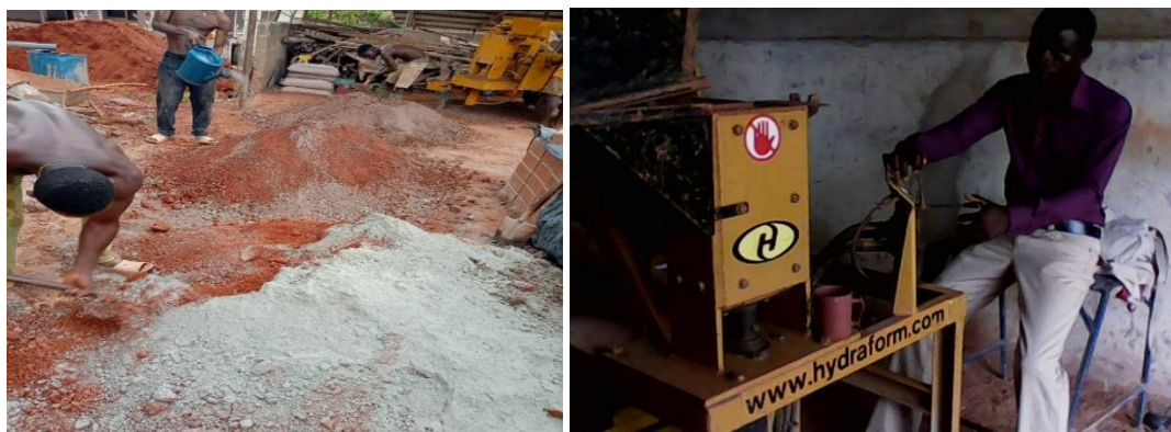
Fig. 6. Mixing and moulding with hydraform machine set up
