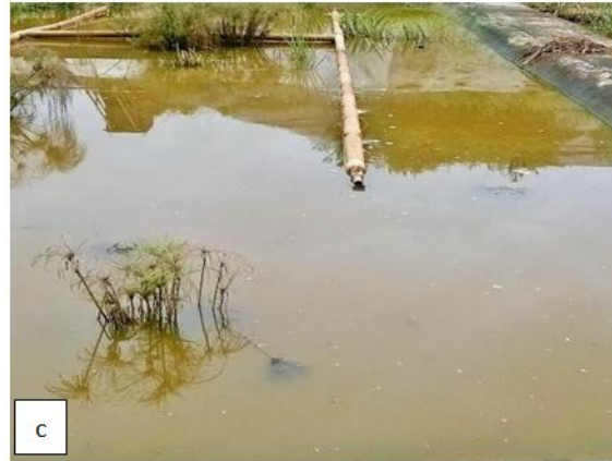
Fig. 8. Progressive disappearance of plants in planted filters: a) PF1 at 1 day b) PF1 at 2 months c) PF1 at 3 months
