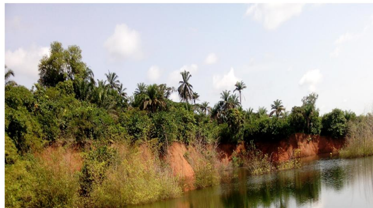
Plate 3. Section of landslide at the river bank
